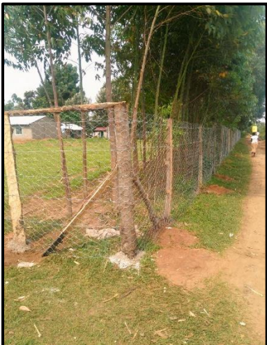
New border fence is being constructed around the School.
